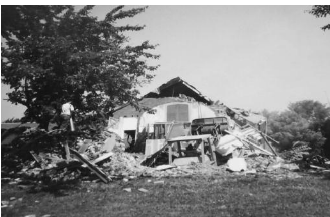
Tearing down old church
