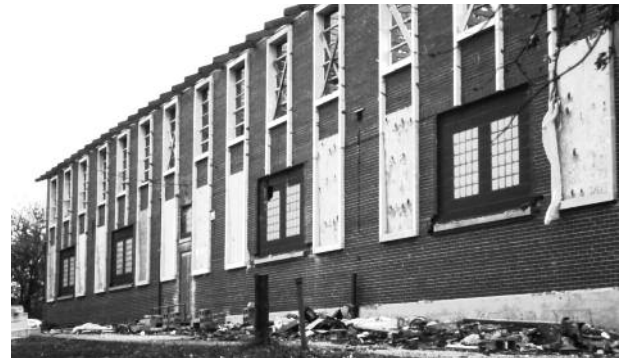
Addition to school 1975
