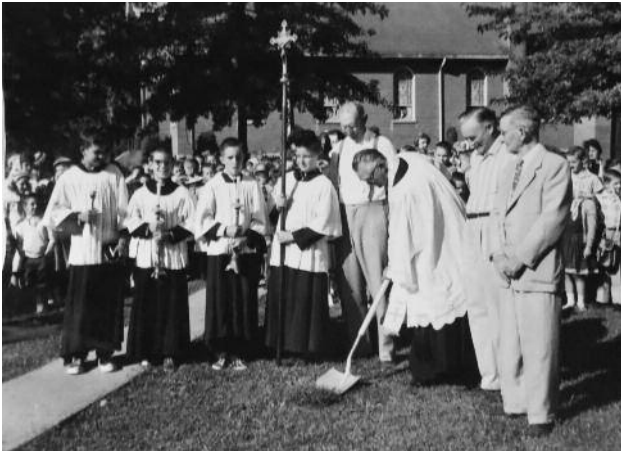
Groundbreaking for church
