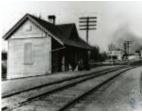
Crescent Springs Train Station
